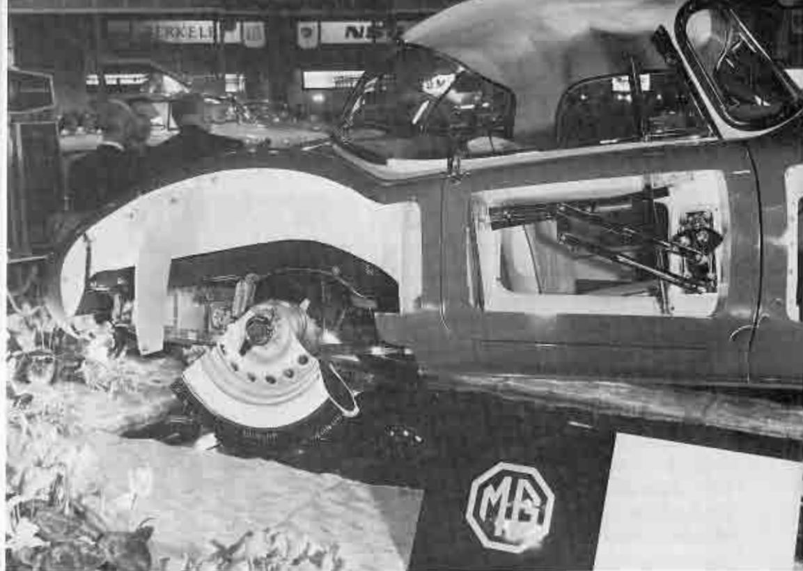
(Above) For the Earls Court Motor show of 1958, MG showed off a partly sectioned example of the MGA Twin-Cam coupe on a revolving turntable. The rear-wheel disc brakes and rear suspension, the window-winding mechanism, and the detail of body roof construction were all displayed to perfection; (opposite) the front half of the same car showed the massive engine, special wheels, Dunlop disc brakes and chassis layout (both Autocar )
