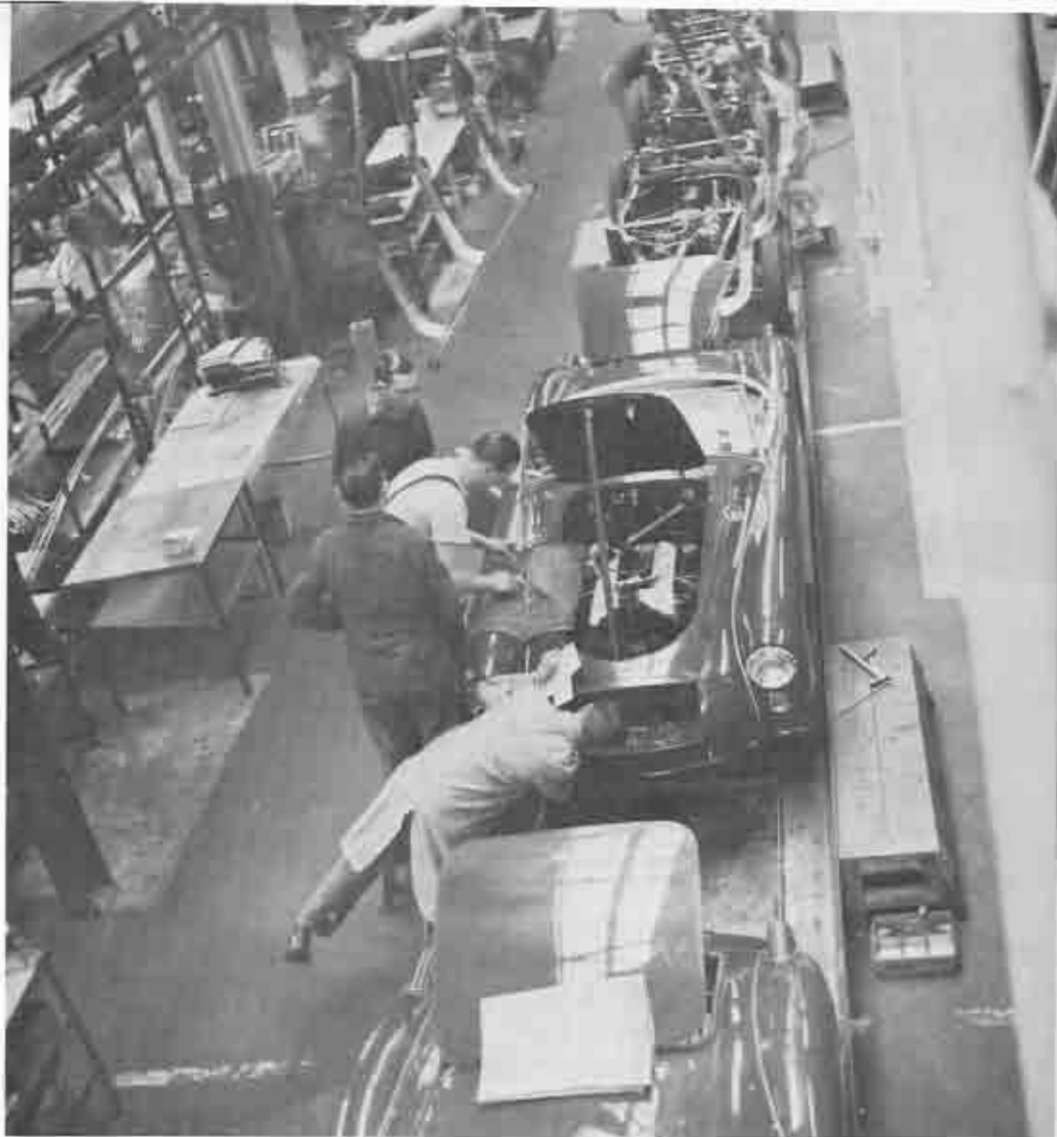
MGA production at Abingdon in 1959/60, with the body of a Twin-Cam just having been lowered on slings to mate with the chassis. Very few Twin-Cams were being built by this stage—all the other cars 'in shot' have pushrod engines (Peter Wood)
